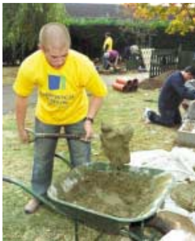
Our partnership with children's charity NCH in the UK provides opportunities for staff teambuilding whilst making a difference to the community, including this garden makeover at King's Lynn, Norfolk.
