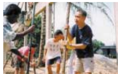
Aviva staff help build the multi-purpose hall for the Orang Asli community in Malaysia.
